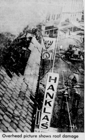
Overhead picture shows roof damage. Fire brought under control after eight hours.
